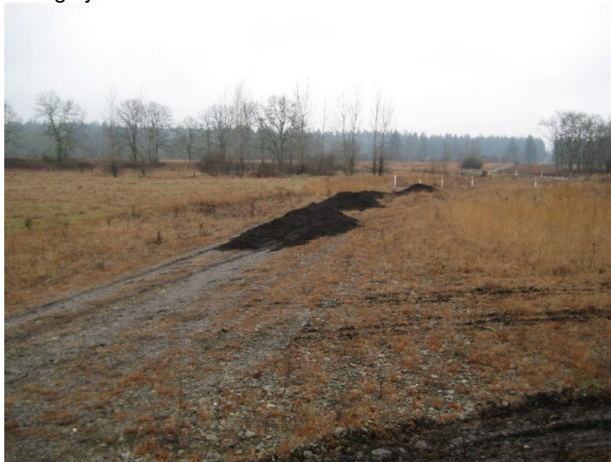
Figure 7: Topsoil delivery at Williams Pipeline restoration site.
