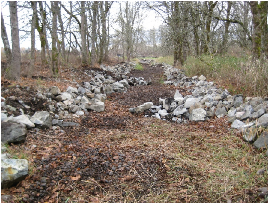
Figure 31: Salmon channel after rock placement.
